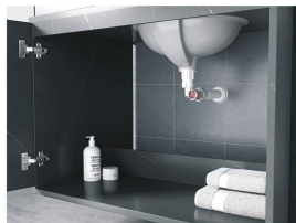
Wall drain 墙排
